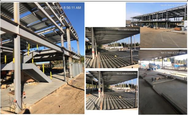
Left to right: Structural steel stairs in place, steel decking for the second floor and roof being set, exterior metal framing, anc concrete pads and footings being poured and set.
