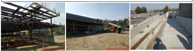
Left to right: Structural steel beams in place (the Canyon Gold signed beam is on the end), steel set for the MPR canopy, ramp handrails being set in concrete base.
