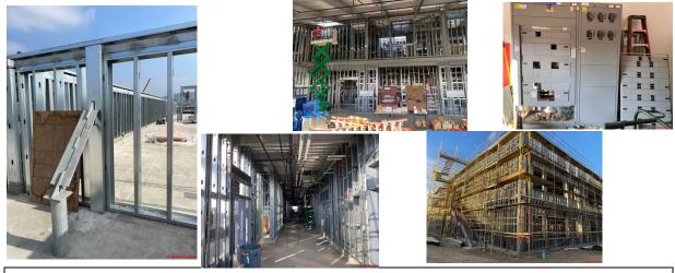
Left to right: Roof top steel framing, interior framing and piping runs (horizontal and vertical), 2<sup>nd</sup> floor framing interior hallway, mechanical bldg.. electrical equipment being set, exterior building scaffolding and stairs.
