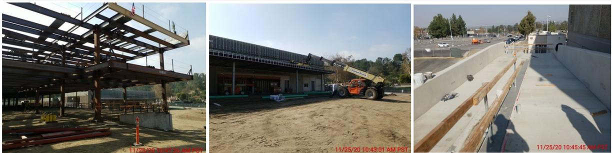
Left to right: Structural steel beams in place (the Canyon Gold signed beam is on the end), steel set for the MPR canopy, ramp handrails being set in concrete base.
