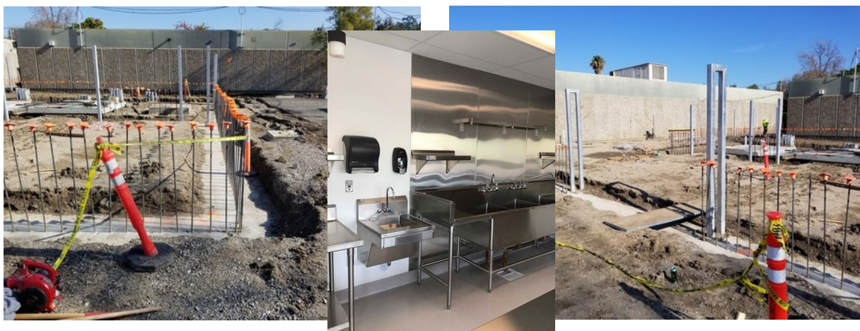
Left to right: Trenching for electrical service yard, Interim kitchen sinks in place including serving line outside, Vertical framing and conduits for the electrical service yard.
