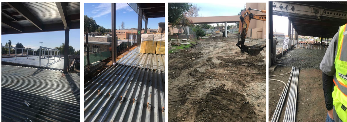
Left to right: Setting steel roof decking with rails and overhang, excavation of main street through campus to Walnut, preparing for conduit interior run and slab pour.
