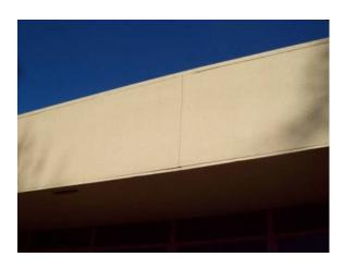
Location:Exterior stucco walls, soffits, and fascia.Material:Plaster SoffitsDistress:DamagedCategory:Deferred MaintenancePriority:3 - Necessary/Not Yet Critical (Years 2-5)Correction:Replace plaster soffitsQty:3,600-S.F.Estimate:\$24,416.64Assessor Name:Ann Buerger LindenDate Created:01/30/2013
