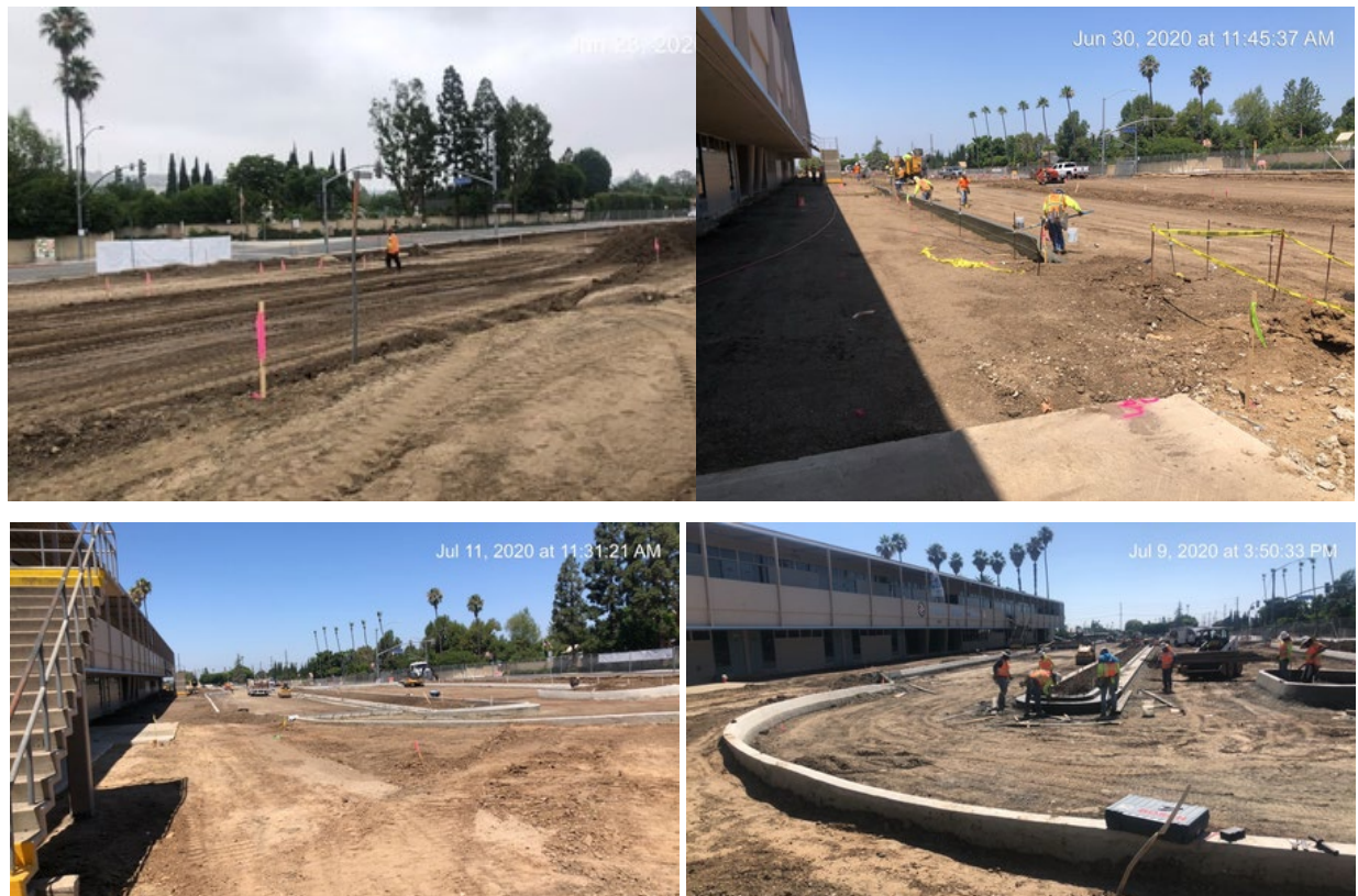
Left to right: Staking, grading, setting concrete pour for curb and middle island for the new drop off area off area in front of the school along Taft.
