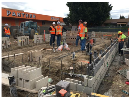
Initial masonry block course for Satellite Kitchen.
