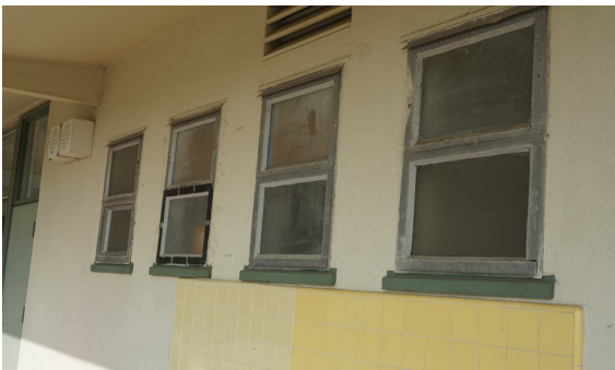
Window thresholds in need of attention.
