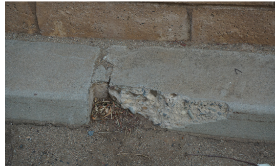
Dilapidated curb condition.
