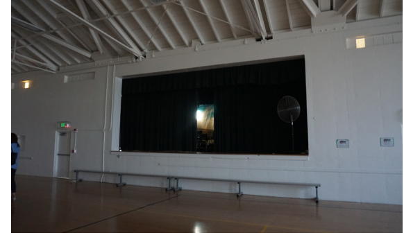
Lack of ADA access to stage.
