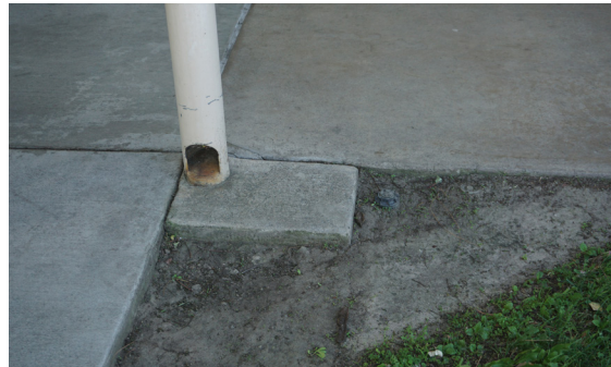
Location of drains causes flooding.
