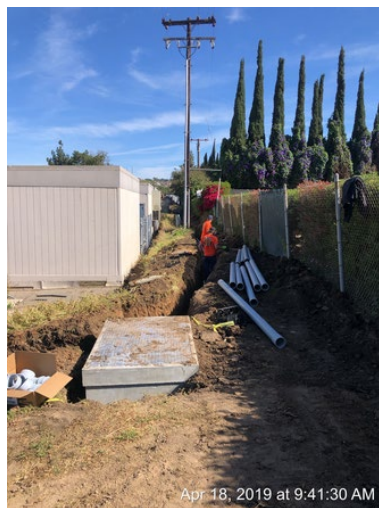
Trenching and setting vault for new electrical power.
