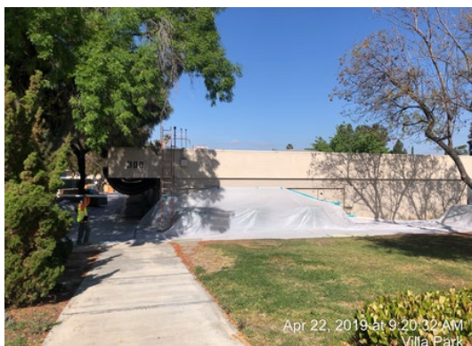
Building 300 in containment for hazardous material removal.
