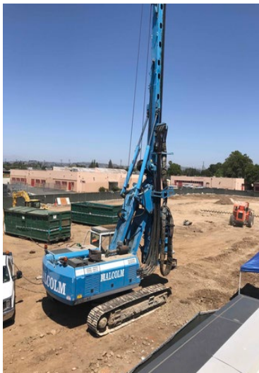
The drilling rig is set for the boring of footings for steel piles at the Science Building.
