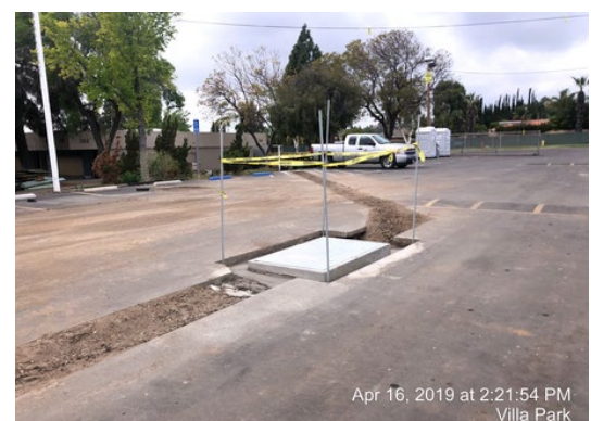
Setting electrical ground vault in place, through the asphalt parking area to the east.
