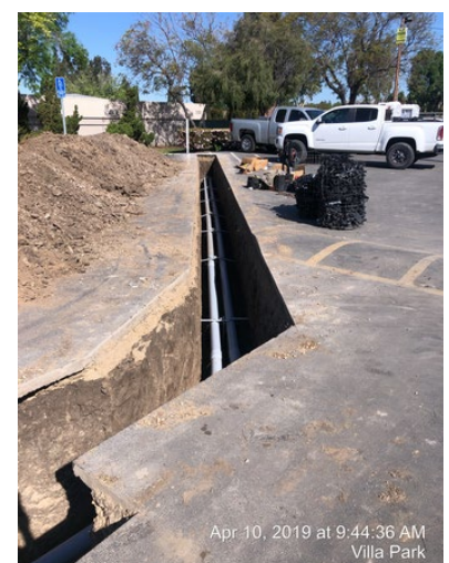
Trenching through the parking area and setting conduits.
