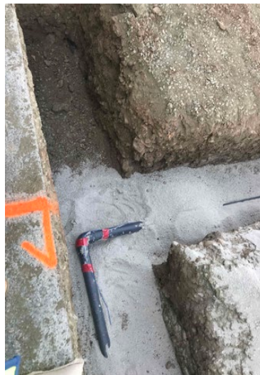
Uncovering and protecting existing piping in the excavation.
