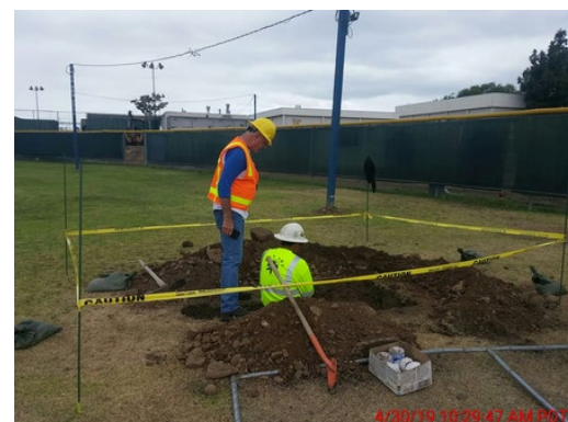
Excavating and uncovering underground lines to be protected.
