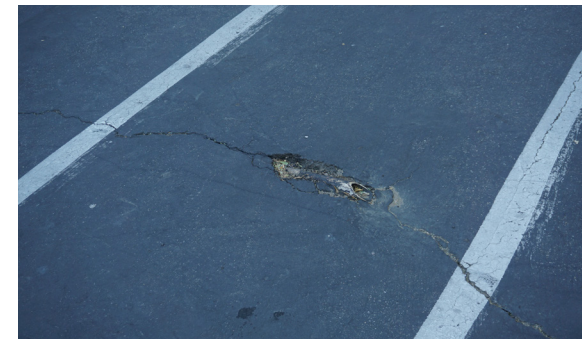
Cracking around hardcourts.
