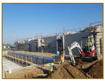
Construction on El Modena High School's Aquatics Center continues at a fast past. Tile is currently being added to the new 30-meter pool. Block construction is nearly complete on the 3,000 square foot locker room/pool equipment building with roof structure installation scheduled to begin in September 2021. The Aquatics Center is on track to open in Spring 2022. The project is being paid for by the District's special capital outlay reserve fund which is funded by the sale of surplus property.
