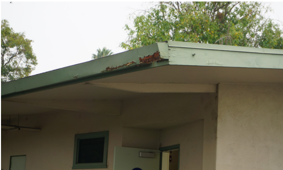
Damaged fascia boards.
