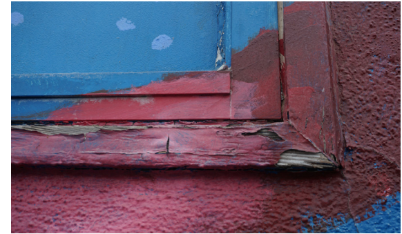
Exterior paint chipping.
