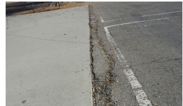
Cracked hardcourt surface.
