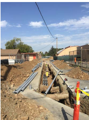
Electrical underground adjacent to building 800 south.
